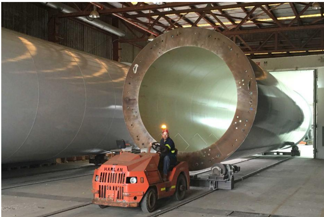
Tower construction at Keppel Prince factory, Portland
